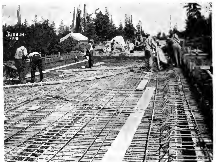
Reinforcement for river bridge, Marine Highway, B. C.
